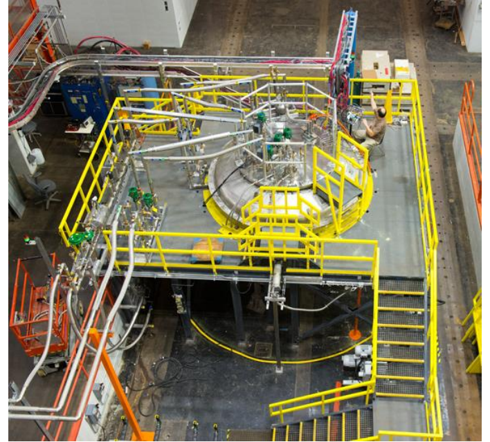
Exterior of the existing Solenoid Test Facility at Fermilab (Image: Fermilab)
