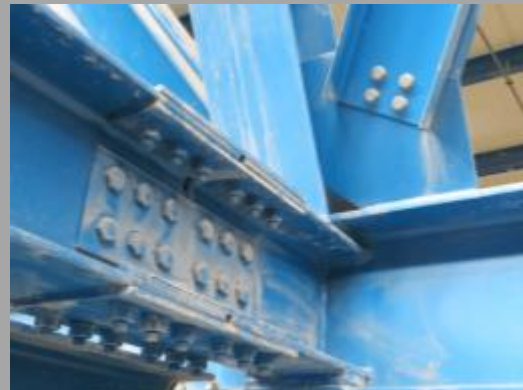
Diagonal trusses from upper to lower spine beams broken (26 out of 32) partly at top, partly at bottom connection plate
